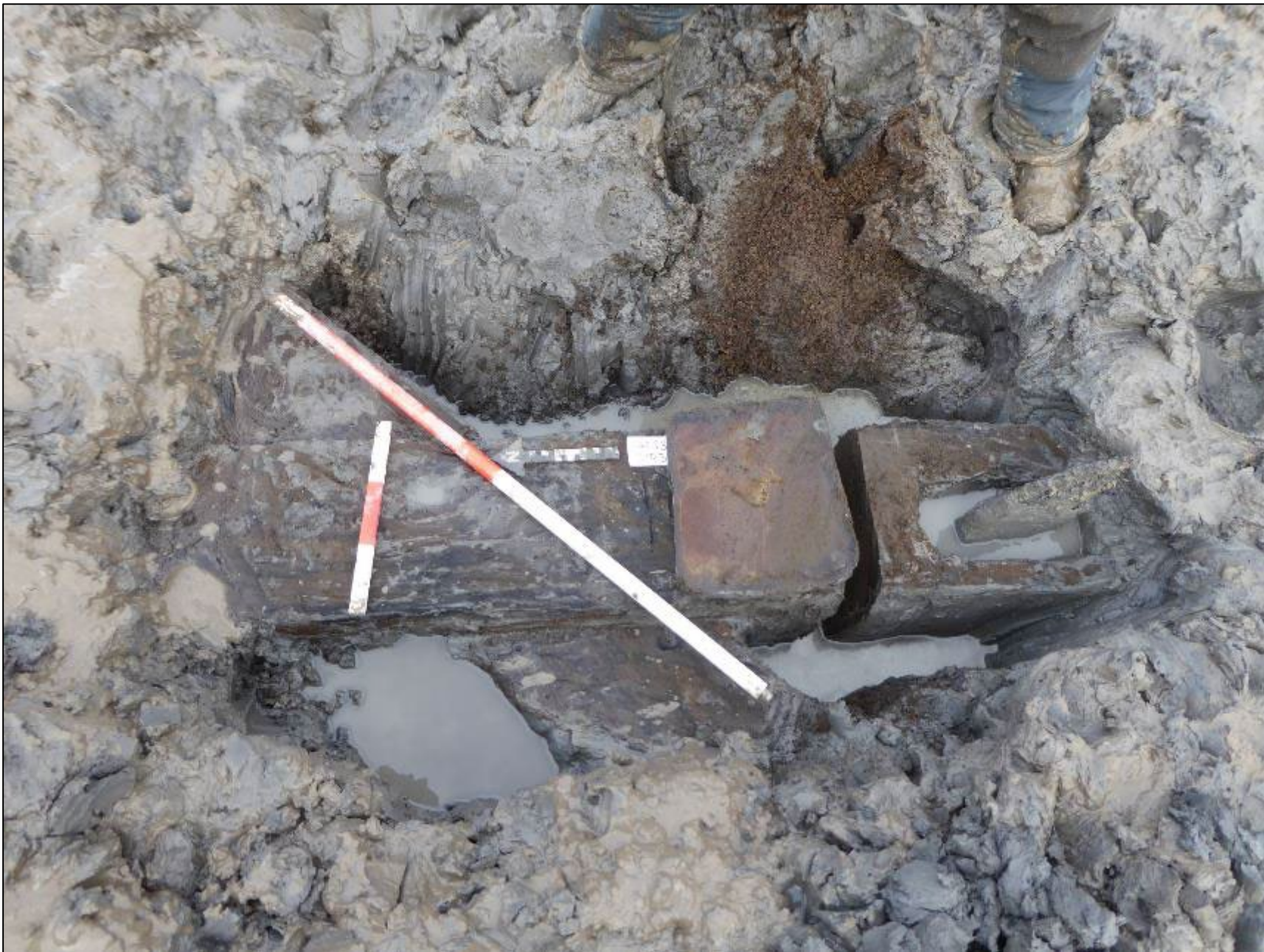
Sample 3. Joint at the downstream end of the structure.
